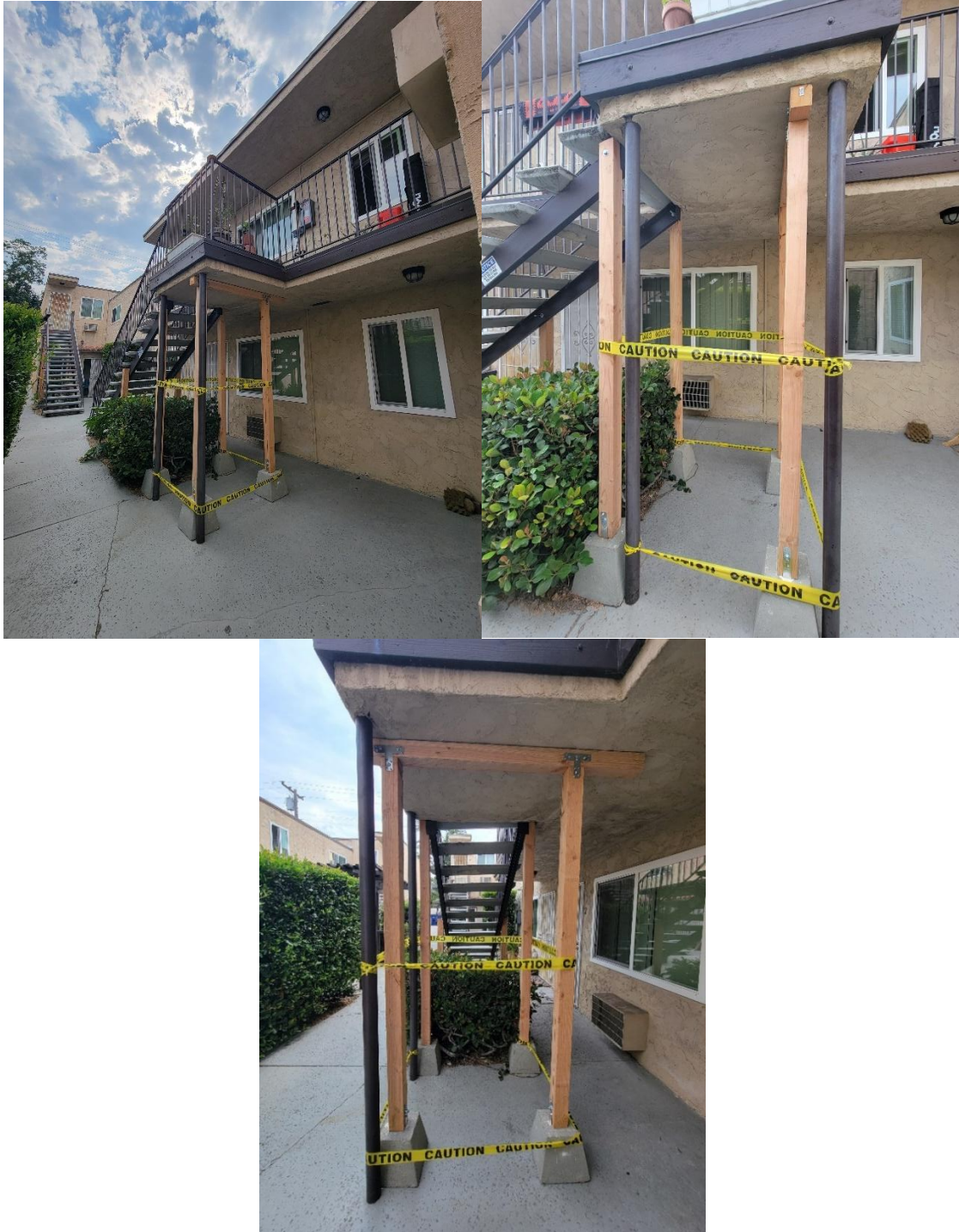
Picture 31: View of temporary shoring including 4x4 beam and posts, and concrete block footing.
