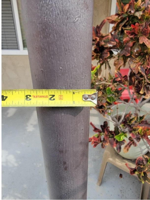
Picture 15: Typical steel tube post measured 3" outer diameter.
