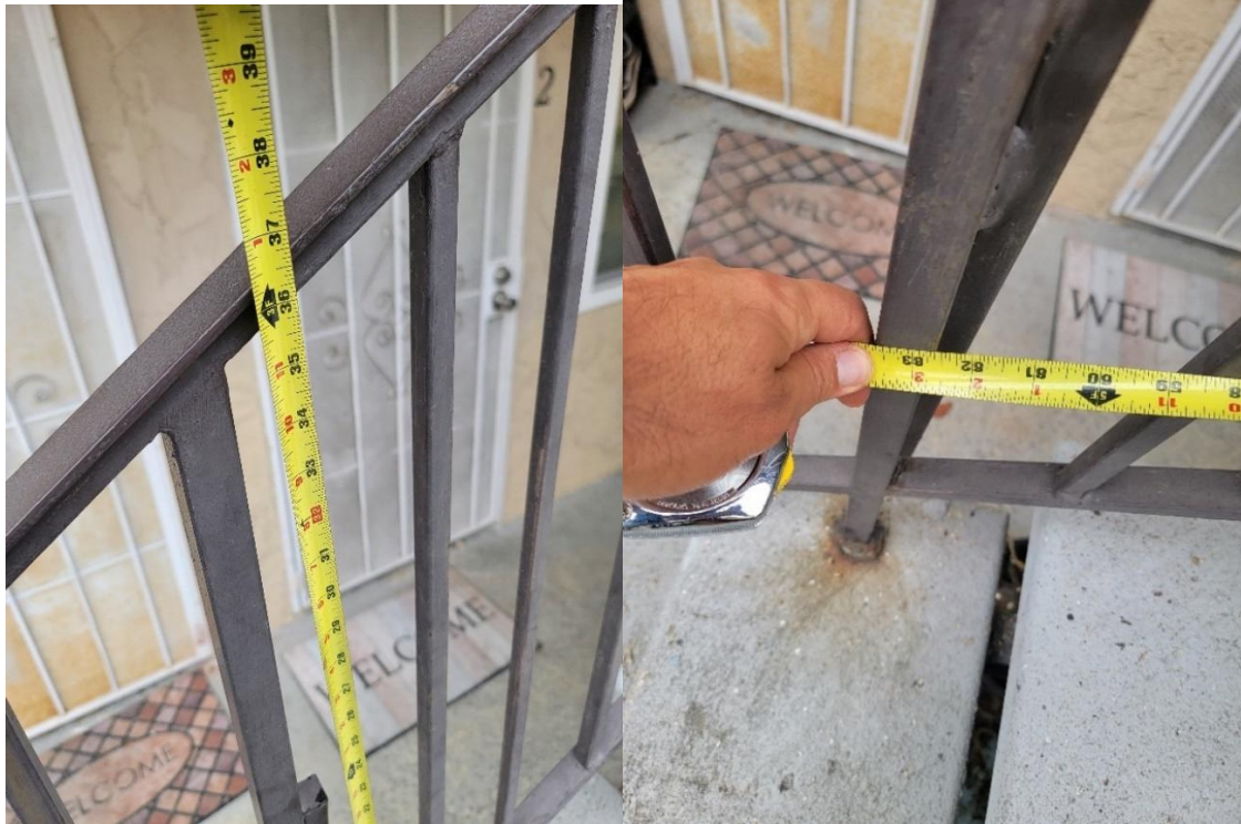
Picture 28: The stair railing is 36" high, post spacing varies with approximately 5 feet 3 inches post spacing on this picture.
