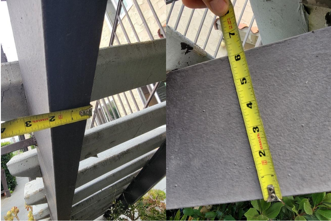
Picture 9: Steel stringers are channel measured 6" deep and 2" flange width.
