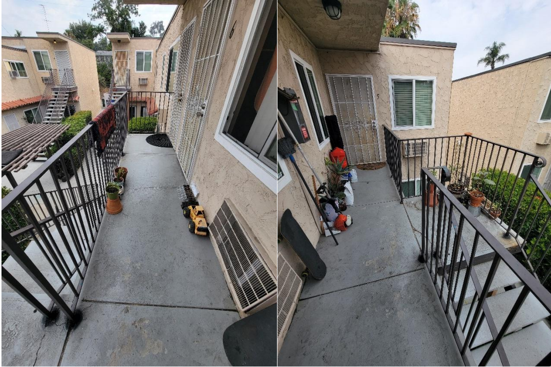
Picture 34: Views of landing and walkway
