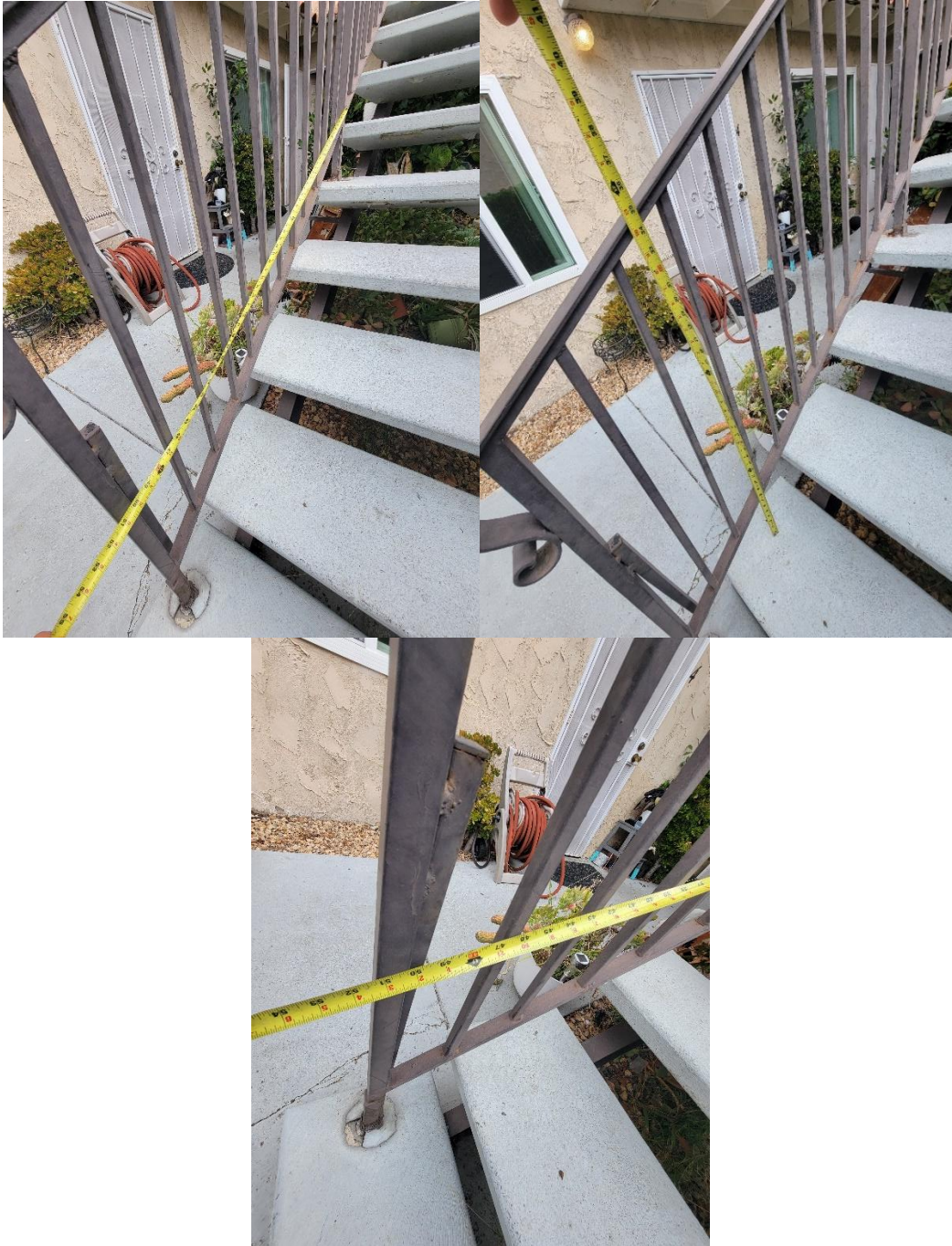
Picture 3: The stair railing is 35" high, post spacing varies with approximately 4 feet 2 inches post spacing on this picture.
