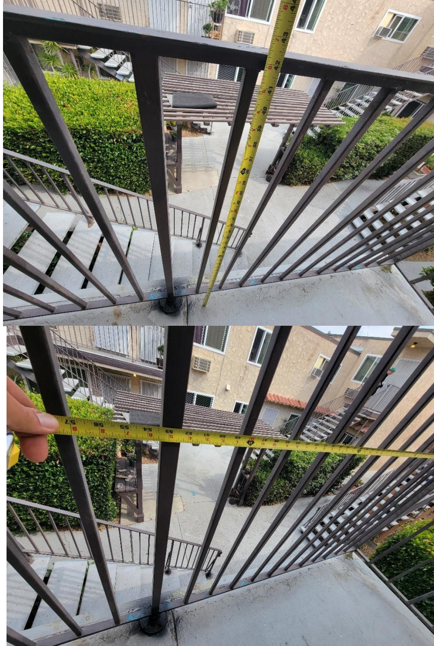
Picture 29: The landing railing is 42" high, post spacing varies with approximately 4 feet 5 inches post spacing on this picture.
