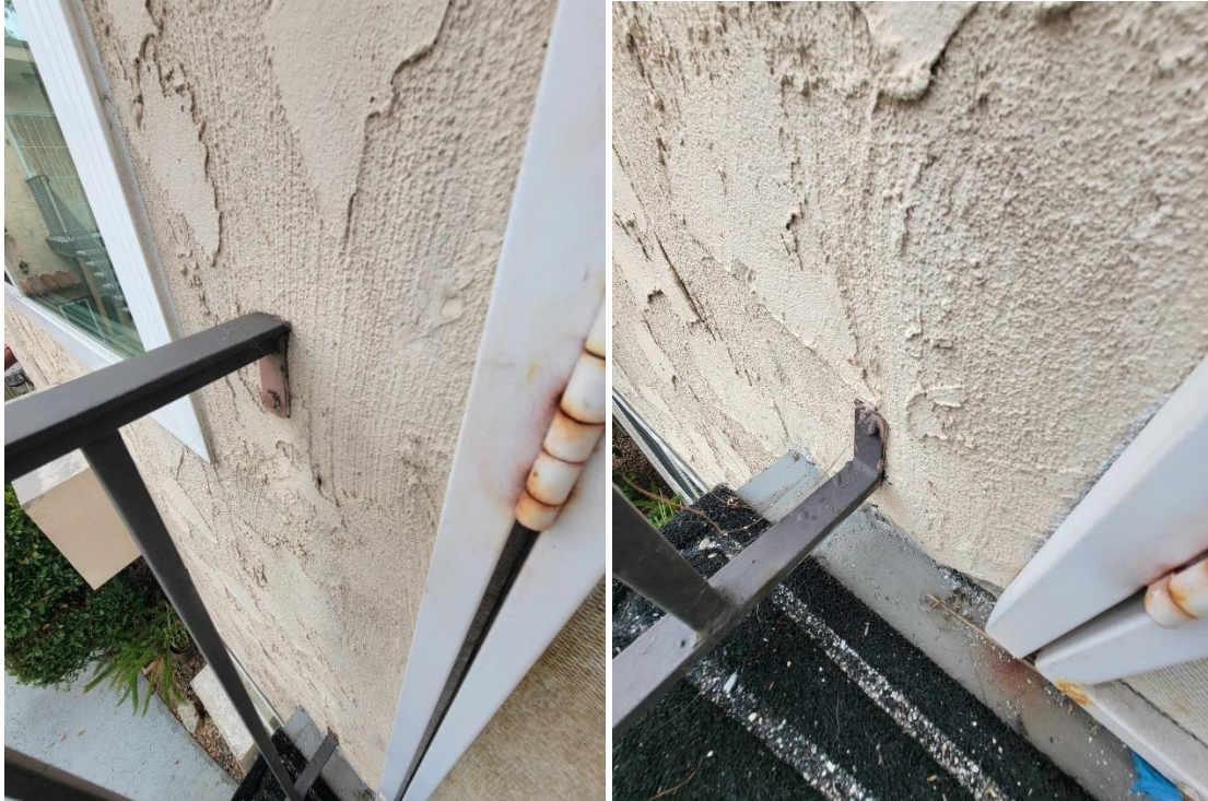
Picture 37: View of the landing railing anchorage to exterior stucco wall
