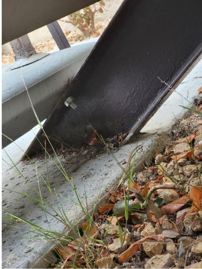
Picture 10: Typical steel stringer connection at the slab on grade
