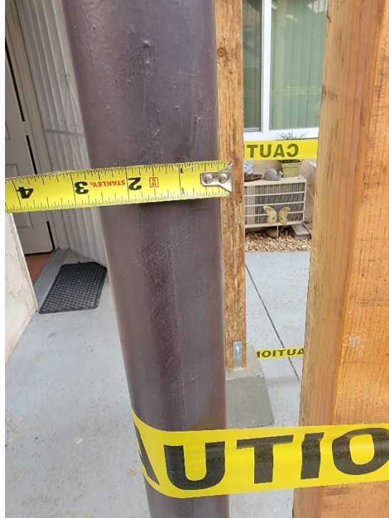
Picture 24: Typical steel tube post measured 3" outer diameter.
