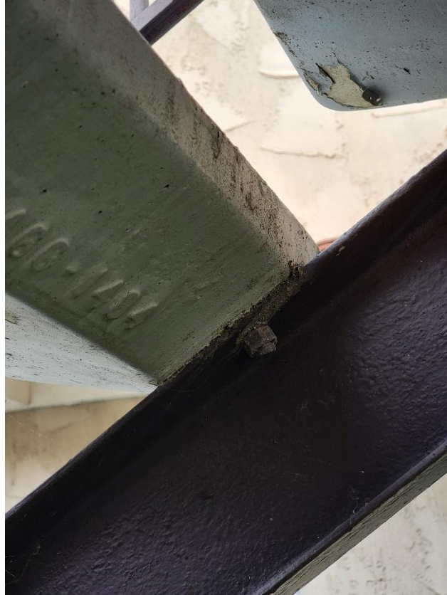
Picture 8: Typical concrete treads bolted connection to the stair steel stringer
