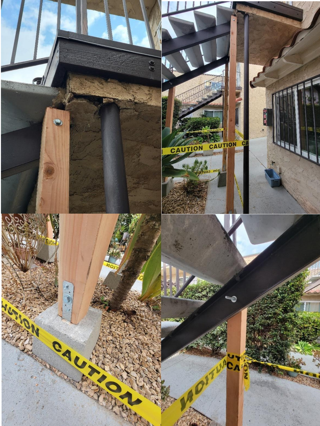
Picture 26: View of temporary shoring including 4x4 posts, block footing, bolted connection to the steel stringers.
