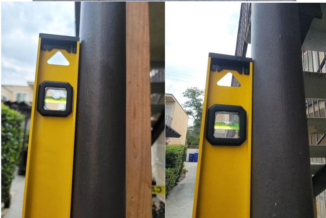
Picture 33: Landing is level, and the posts are vertically aligned “plumb”
