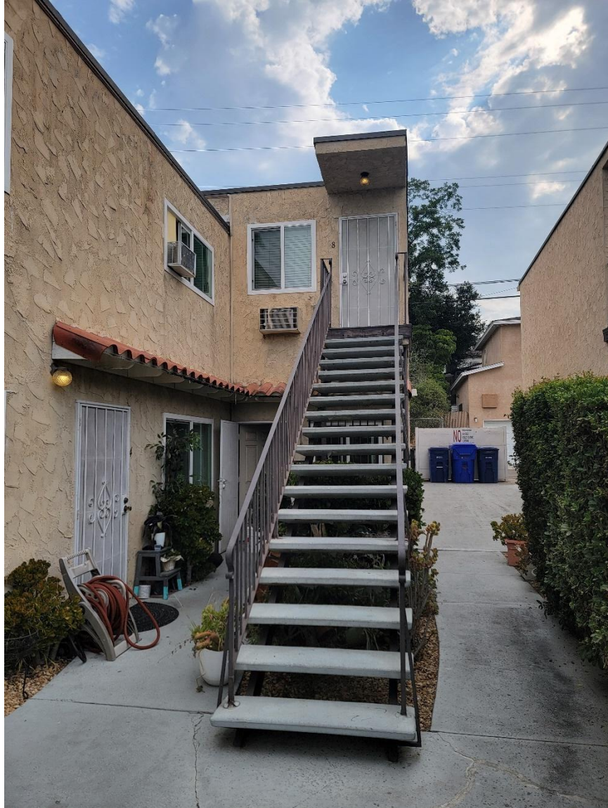
Picture 2: North stair at 4659 3 rd street.
