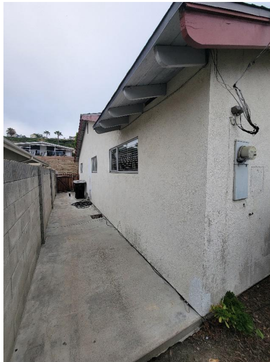
Picture 8: Southwest view of the house
