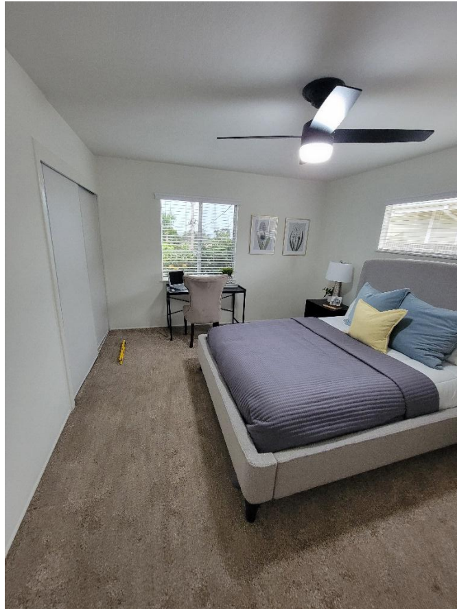
Picture 22: House slab on grade is not flat sloping near south wall towards the foundation potentially due to foundation settlement
