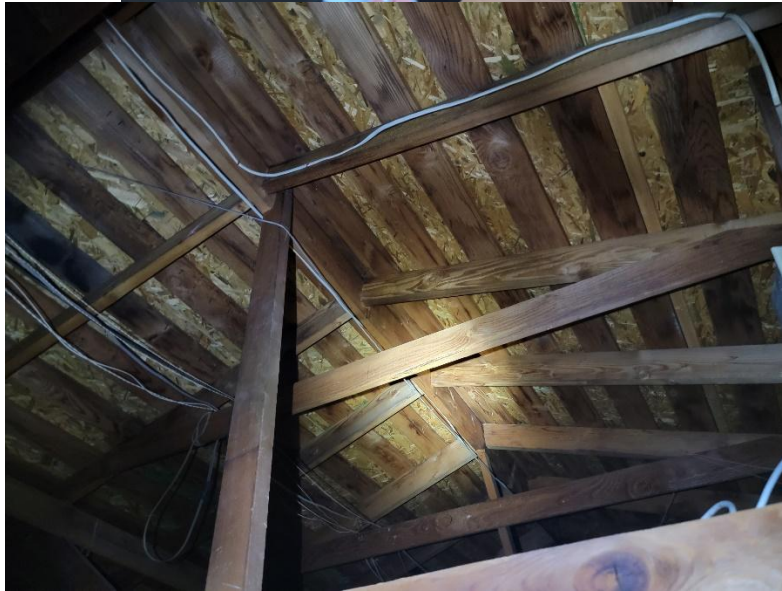
Picture 9: View of the roof wood framing from the attic
